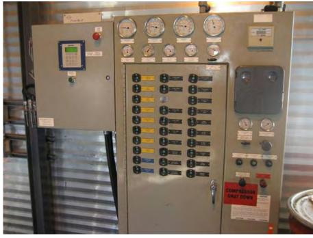
Existing pneumatic control panel with compact DE-3000 panel mounted on left side.
